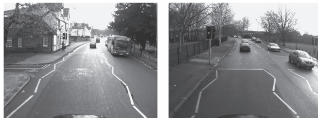
Fig. 2. Zig-zag approach road markings lead up to a traffic light controlled pedestrian crossing.
